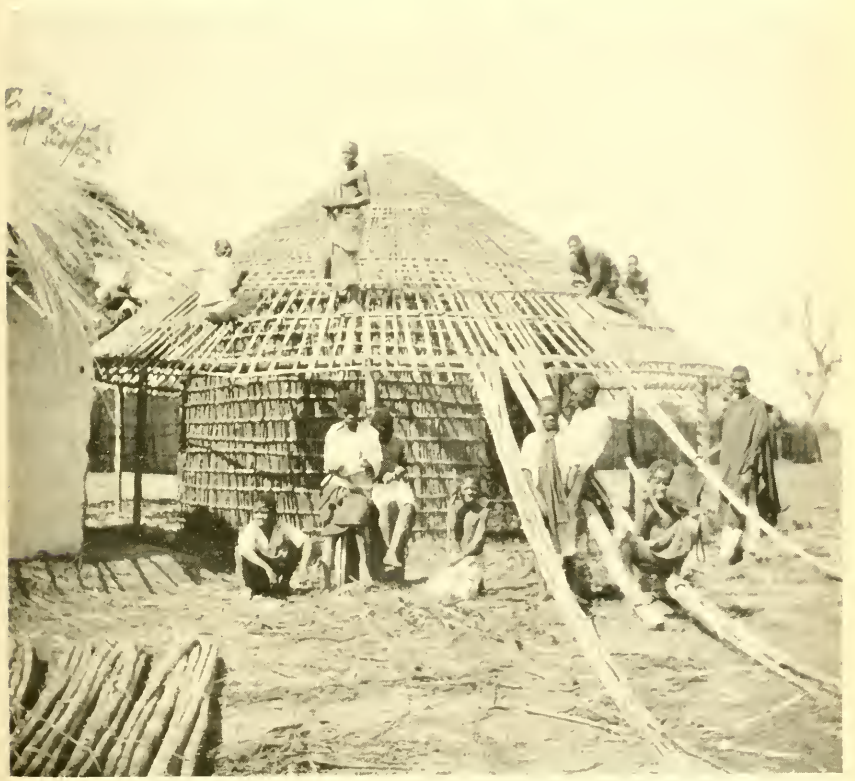
I. FIXING THE POLES. 2. CIRCLE OF SPLIT BAMBOOS, WITH HORIZONTAL CANES. 3. ROOF OF PALM STEMS WHICH IS GRASS THATCHED.
